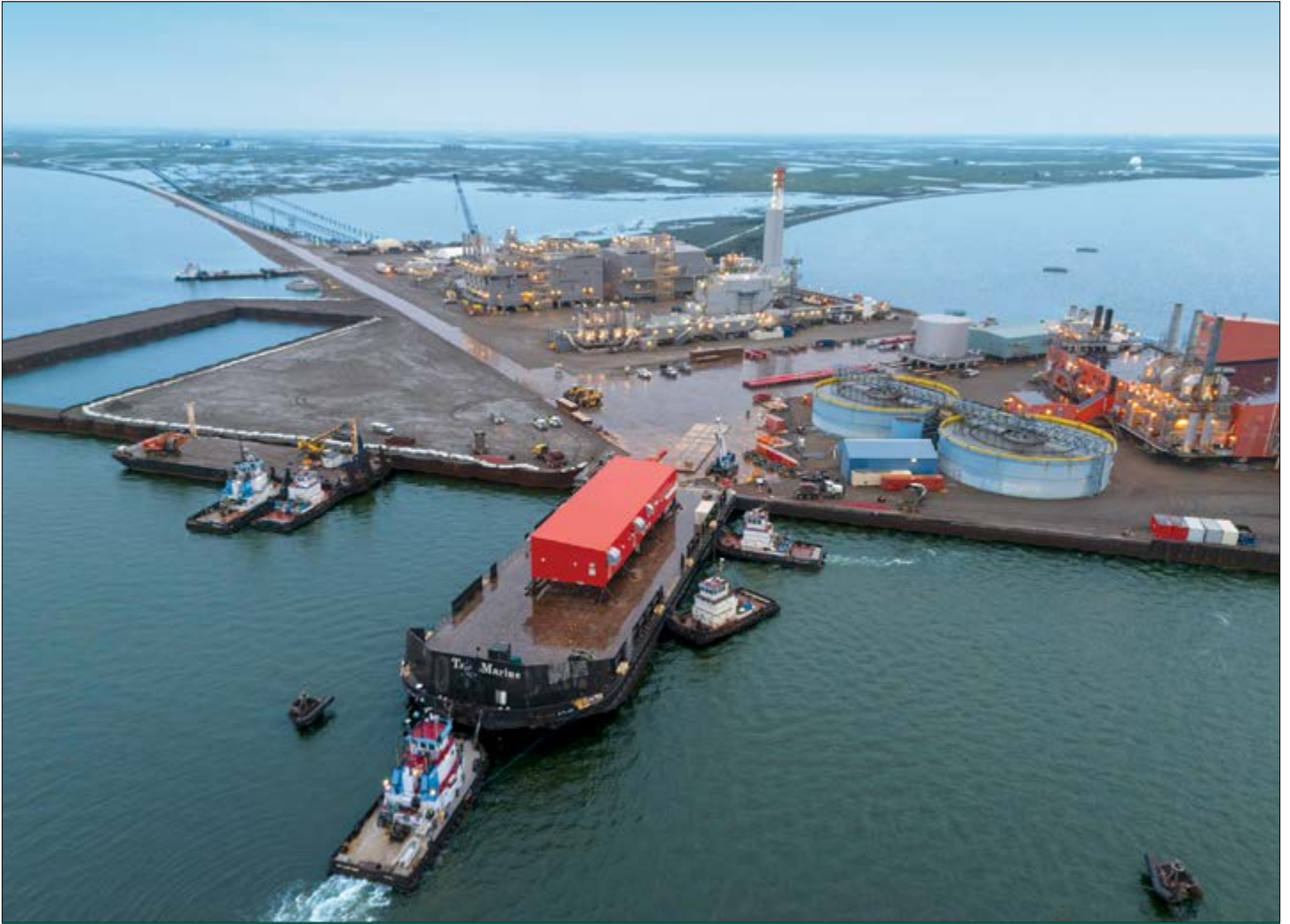
ConocoPhillips' production module for its Nuna project being delivered to Oliktok dock.
