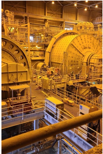
Milling Optimization Project at FK
