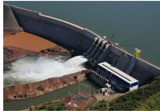
Brazil – two hydroelectric power plants with 155 MW capacity
